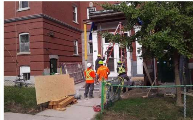
REPAIRS ARE UNDERWAY
